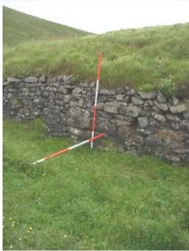
Figure 8: H2 viewed from north west
